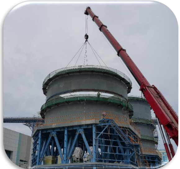
Tank Shell Erection
