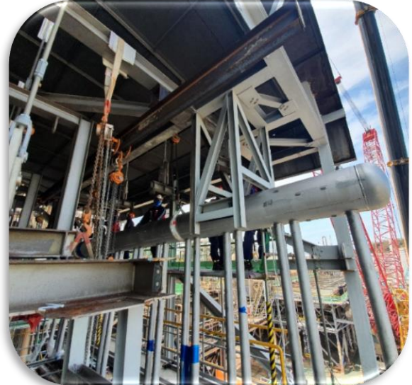
Heater Coil Install
