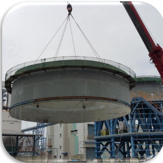
Tank Shell Erection
