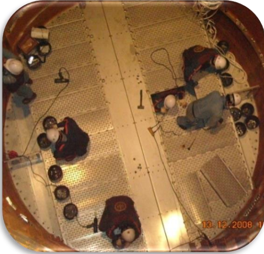
Column Internal Install
