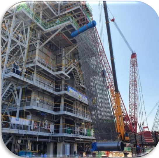
Heater Coil Install
