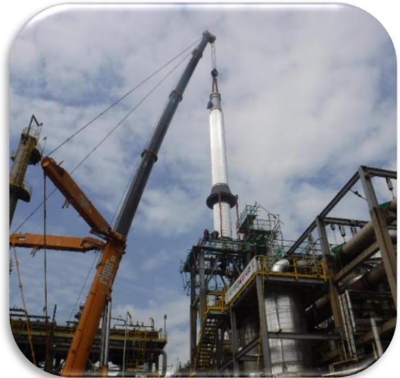
H/Exchange Install
