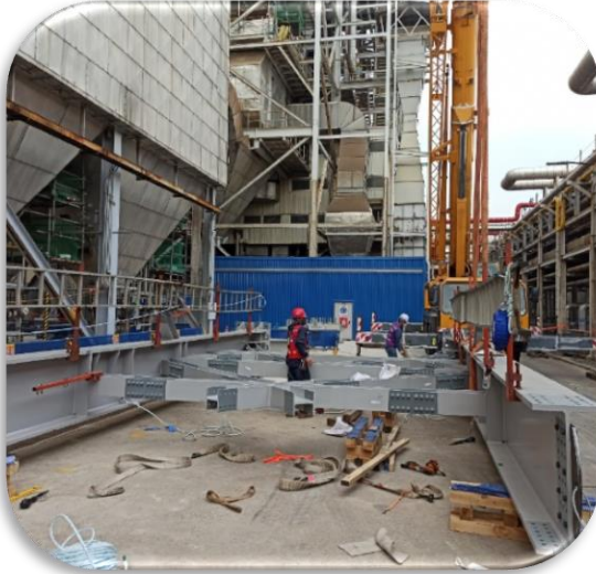
STR. Field Erection
