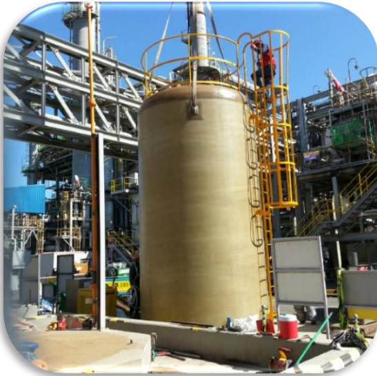
FRP Tank Install
