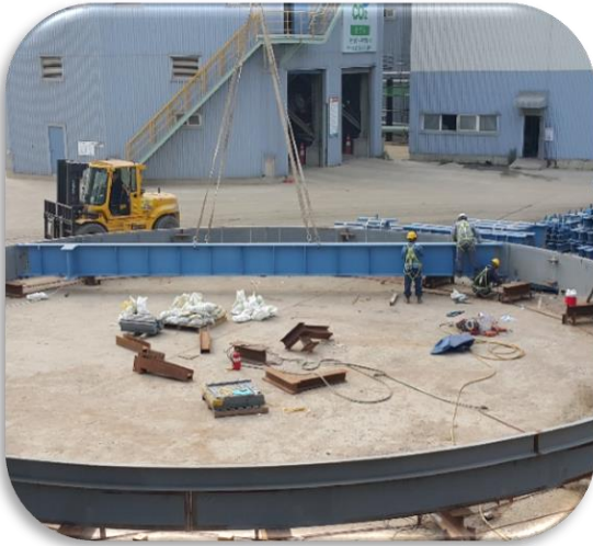
Tank Fabrication
