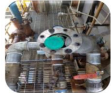
Metal Pin Pig mounting
