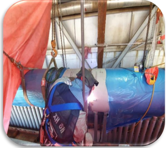
Coil Header Welding
