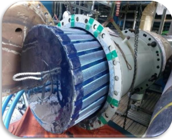
Line Pig Cleaning
