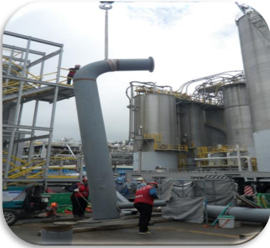
Pipe Erection
