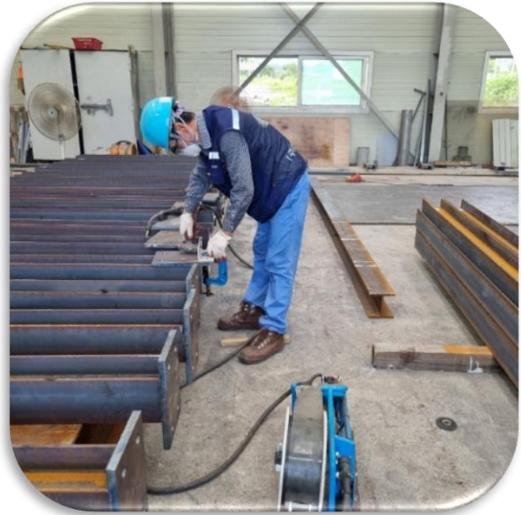
STR. Shop Fabrication
