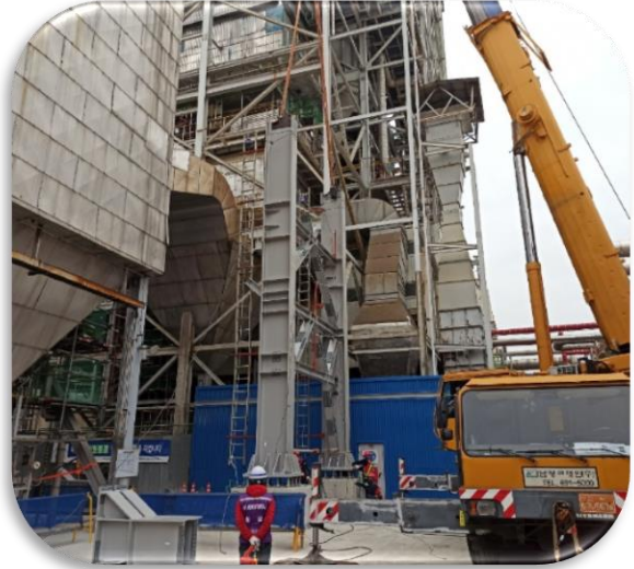
STR. Field Erection
