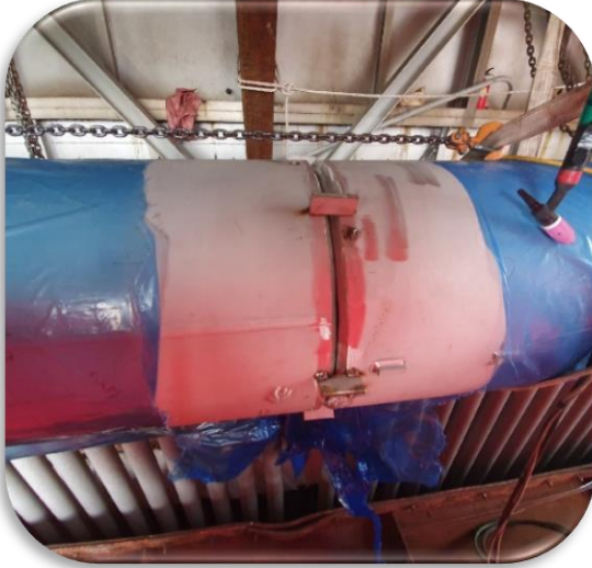
Coil Header Fit-Up
