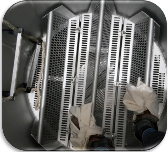
Vessel Internal Install
