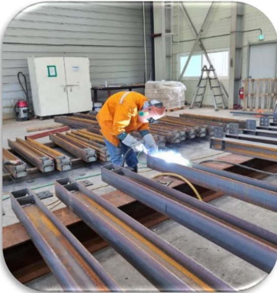
STR. Shop Fabrication
