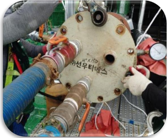
Line Pig Cleaning
